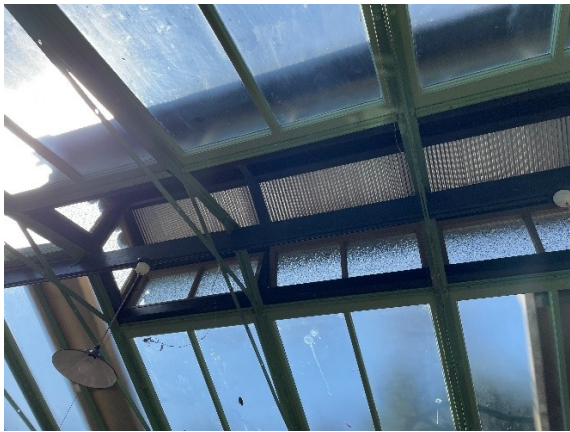
Cantilever roof opening
